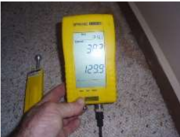
23. In the rumpus room all along the West wall & the South wall I got significantly elevated moisture readings. Here I am showing the moisture meter with a reading of 129.9.
