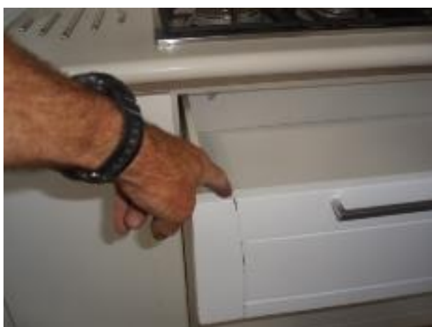
44. The drawer front has had a knock & the damaged portion glued back on.
