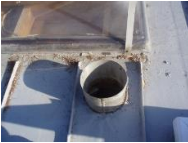
17. The disused flue.
