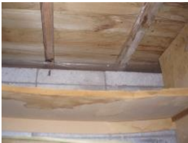
41. Another view of the cupboard ceiling.
