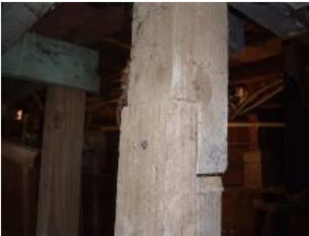
34. The subfloor space.
